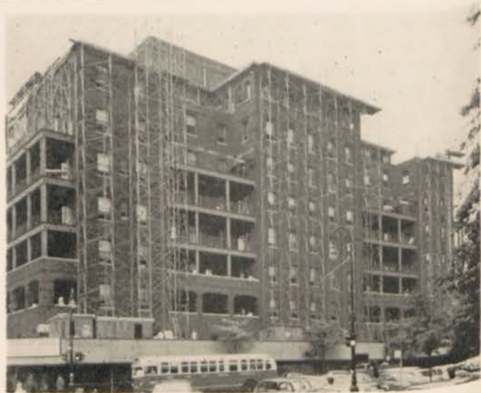
SCAFFOLDING ON FRONT OF HOSPITAL MADISON AVENUE SIDE
