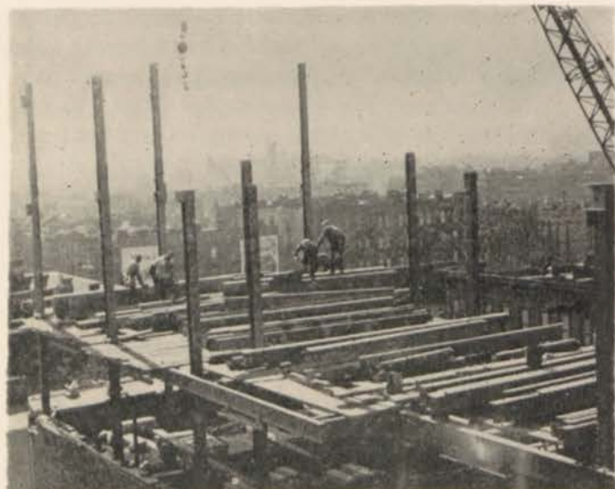
NEW FLOORS BEING ERECTED ON OUT-PATIENT BUILDING
